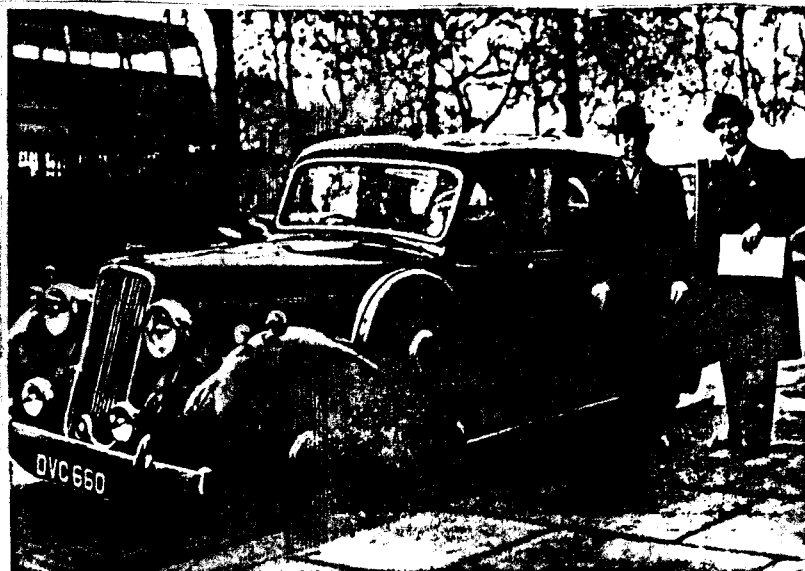
73A: Humber Pullman had same 4085.7-cc six-cylinder engine as Super Snipe and Imperial but 11 ft wheelbase. Shown is a Limousine by Thrupp & Maberly.
