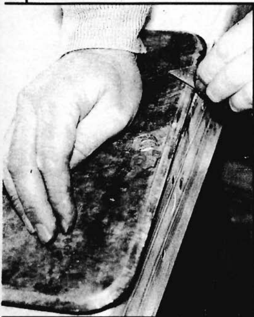
211 First stage of woodwork renovation is to remove all old varnish. After using Nitromors as explained in the text the old varnish is scraped off. Geof finds it best to scrape towards him – the blade tends to jump if pushed away.
