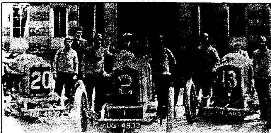
The 1914 TT Humber team, L to r: Sam Wright's car (No. 20); Burgess' car (No. 2); Tuck's car (No. 13). The different cross-member/starting-handle configuration on Tuck's car can be clearly seen.
