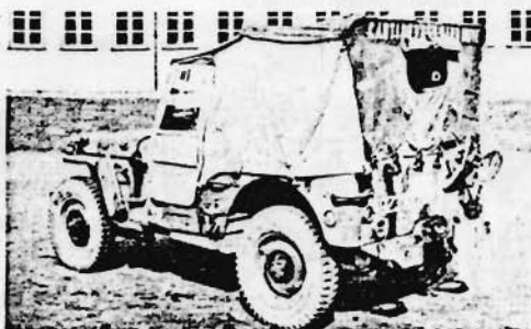
Car, 5-cwt, 4x4 (Willys MB) This was the nomenclature by which the 1/2-ton 4x4 'Jeep' was known in Britain. Shown is an early Willys fitted with all-weather equipment, made by Humber Ltd in April, 1944. British fitted sidelights on front wings (fenders).
